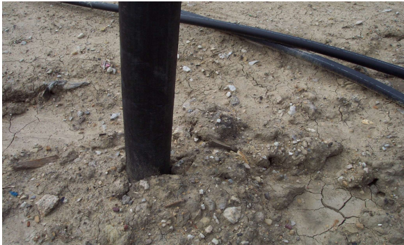
Vertical Landfill Gas Extraction Well
