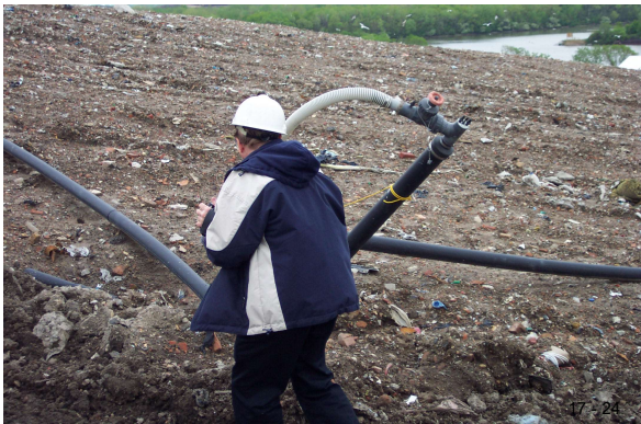
Landfill Vertical Gas Extraction Well
