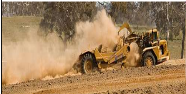
Building New Sections/Cells at the Landfill
