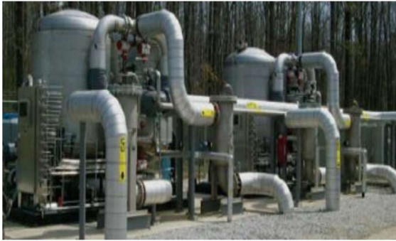
Siloxane removal systems at the Lorraine power station at Oberlin, Ohio
