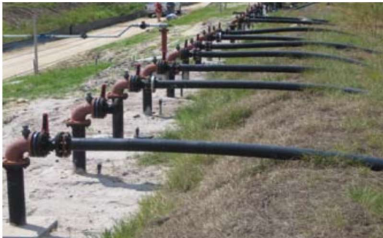
Leachate Injection Pipes
