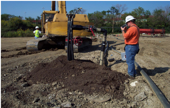
Combination Extraction Well at Landfill
