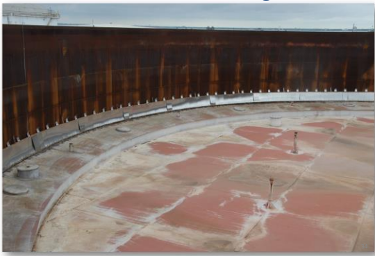
Pontoon Steel Floating Roof
