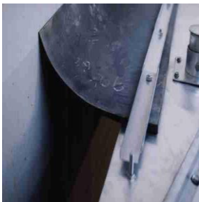
Vapor-Mounted Wiper Primary Seal
